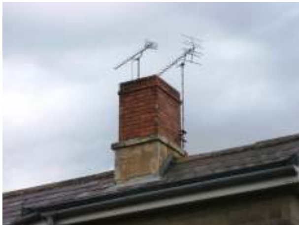
Rear view of chimney stack
