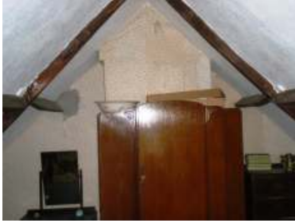
Partially exposed roof structure in attic
