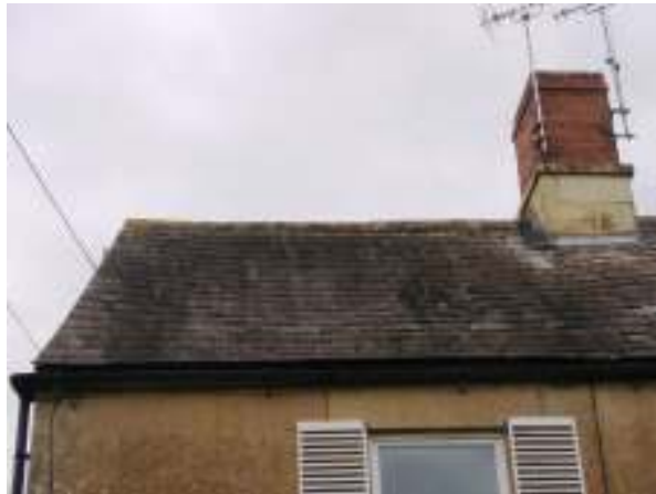
The front roof slope
